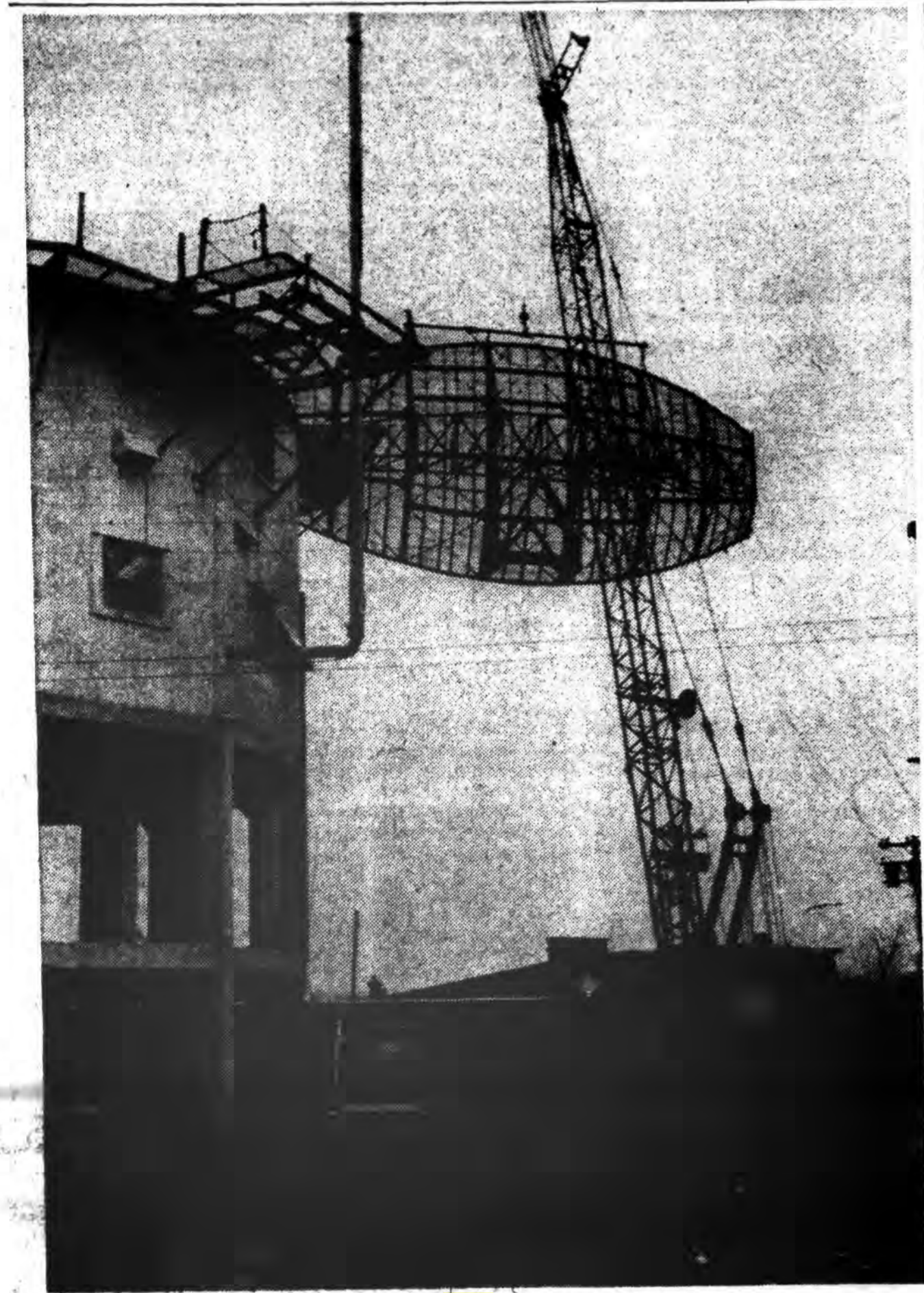
ENLARGED AIR PROTECTION —The radar unit charged with sweeping an assigned vector of sky at the 656th AC&W Squadron, U.S. Air Force, Saratoga Springs is getting a "face lift." The hard rubber dome which covered the unit was removed, the old radar "sail" taken down and replaced with this newer, larger model which will be covered with the latest innovation for radar domes, a rigid model, built of plastic sections. The main purpose of the dome is to protect the sail from weather.
