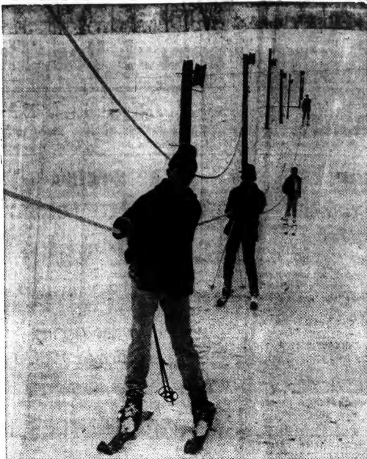
NIFTY LIFT —This 800 foot long ski lift was put together from salvaged materials by men stationed at the 656th Radar Squadron, Saratoga Air Base. The pulleys on the poles are auto wheel rims from a junk yard and an old abandoned car provides the power. Seen coming up the slope are Pvt. Frank Allen and Mike Mac Monagle. Lt. Eaton Laitinen was the project officer in charge of developing the facility and he was assisted by volunteers from the Squadron. Edward Taylor of the Alpine Ski Shop in Saratoga Springs offered advice.
