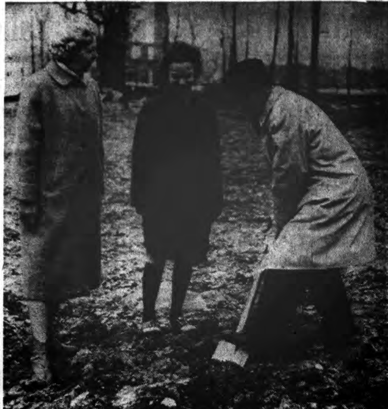
LIBRARY STARTED — Beginning of the first academic building at the new Skidmore College campus was marked when President Val H. Wilson recently turned the ground for the new Lucy Scribner Library. Witnessing the groundbreaking were Skidmore Librarian Gladys M. Brownell and Miss Marilyn Goldstein '64, chairman of a student library committee. The construction contract, awarded to Wade Lupe Company of Schenectady, was signed yesterday. The library is to be completed by August 1965.
