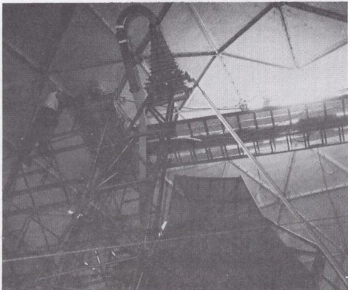
Inside the FPS 26 tower the first piece of the dome is removed by the 485th EIS from Griffiss AFB. The glow of light in the picture is the sun coming through.
